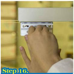
Step 16. Close the door. Make sure the position of strike plate is right and then screw the short U-bracket on door (Including strike plate and plug box)
