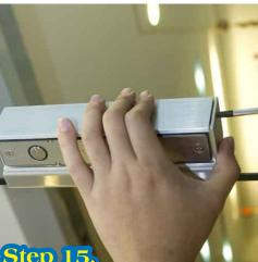
Step 15. Screw the side cover on long plug box
